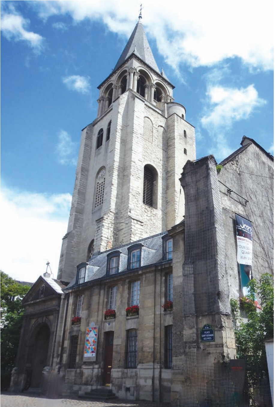
Fig. T2.3. Saint-Germain-des-Près: 1014 bell tower with 19C crown, 1606 outer doorway and 18C presbytery in the foreground.
